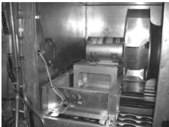
Figure 30 - 9-25 and 30 ton Supply Fan
